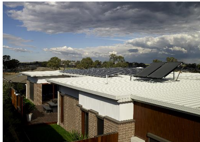
Figure 1: Zero Emissions Home with rooftop solar PV and solar hot water.
